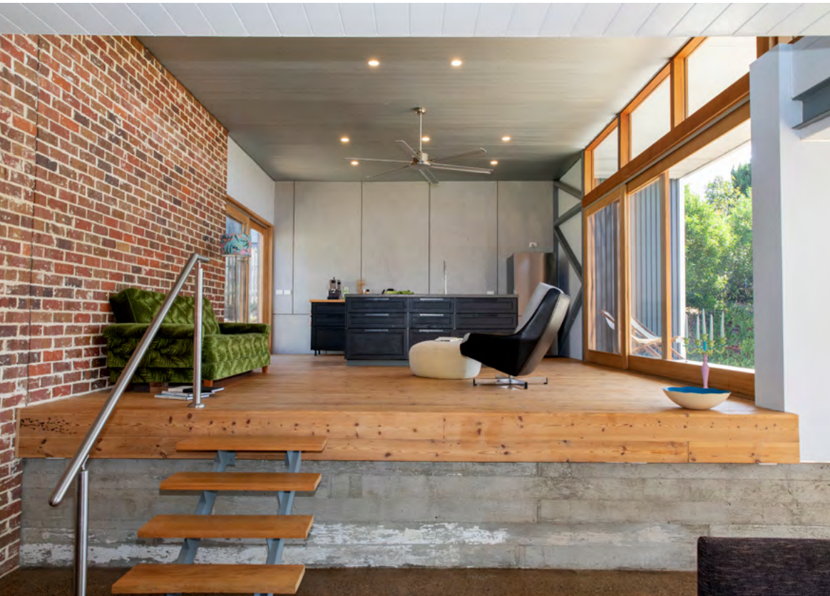
← An insulated recycled brick wall adds to the thermal mass provided by the concrete slab floor to the lower part of the house.
